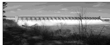
Clarks Hill Dam (1954)
