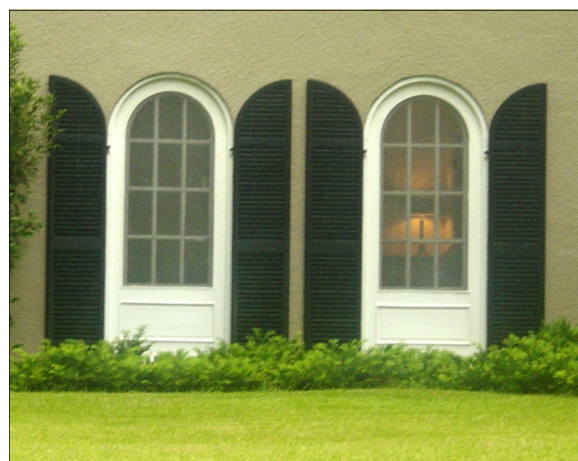
Arched Windows w/ Louvered Butterfly Shutters (Note: will cover entire window when closed)
