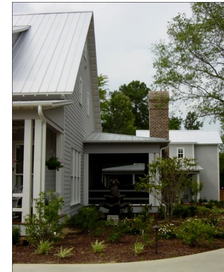
Side Screened Porch
