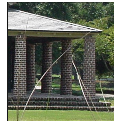
Round Tapered Brick Columns
