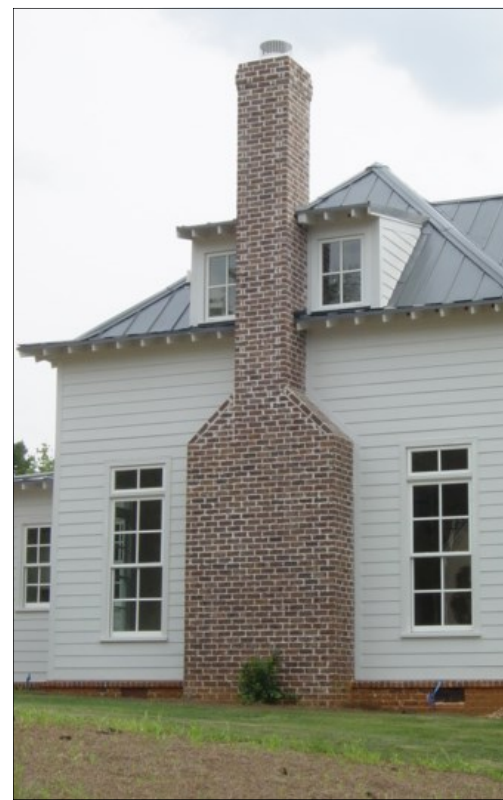
Brick Chimney and Foundation
