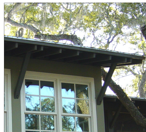
Exposed Rafter Tails with Bracketed Cornice
