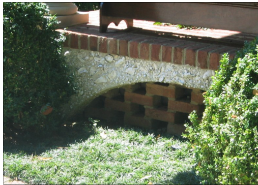
Tabby Foundation w/ Pierced Brick Detail
