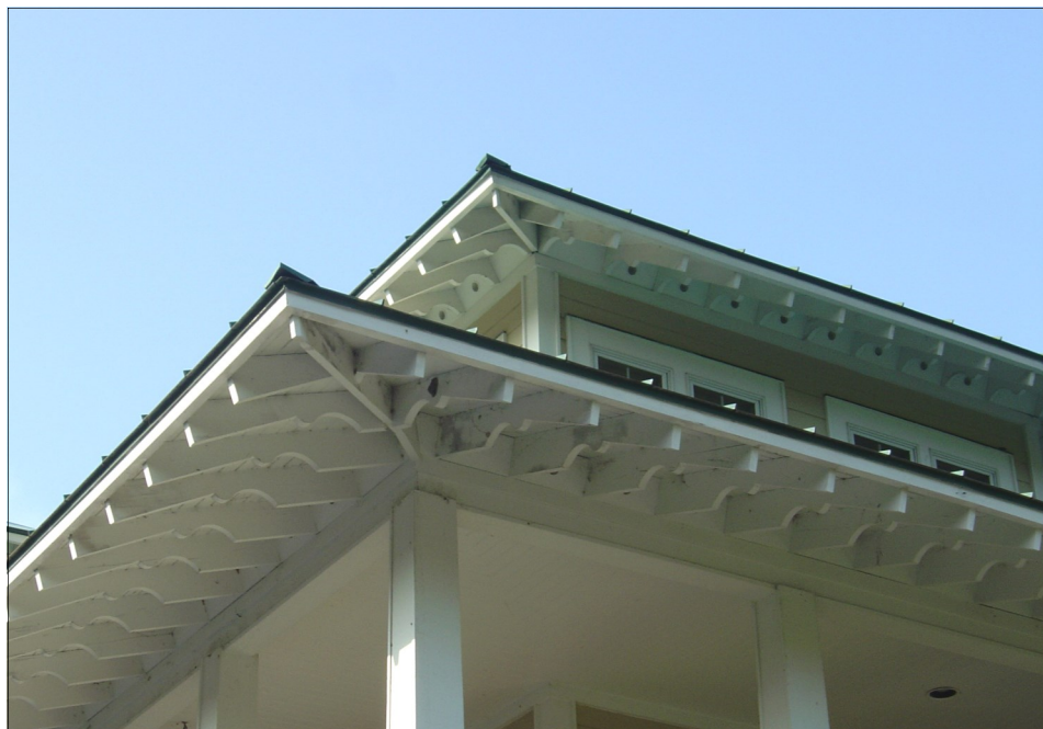
Exposed Cornice with Exposed Rafter Tails
