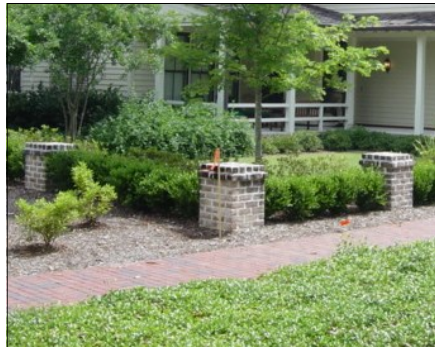
Hedge Fencing with Brick Pilasters
