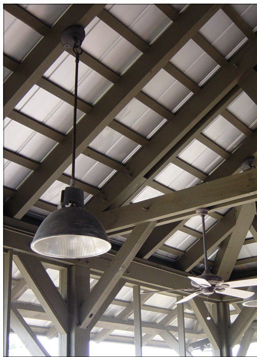
Exposed Metal Roof
