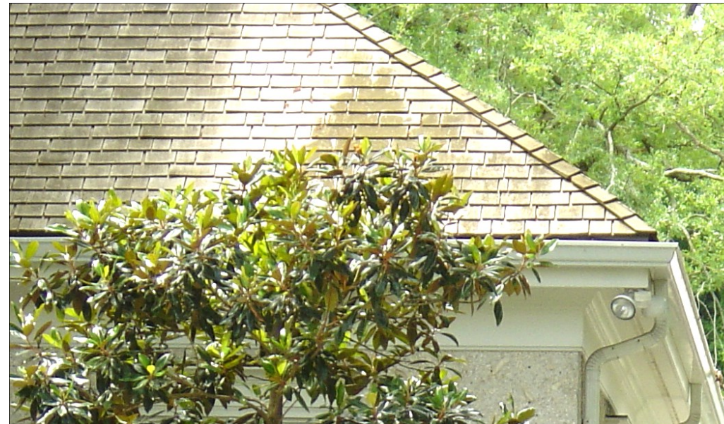
Shake or Shingle Roof
