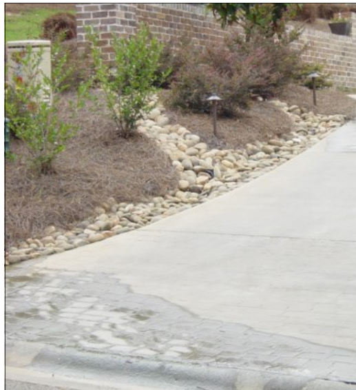
Concrete Drive with Stone Run-off System
