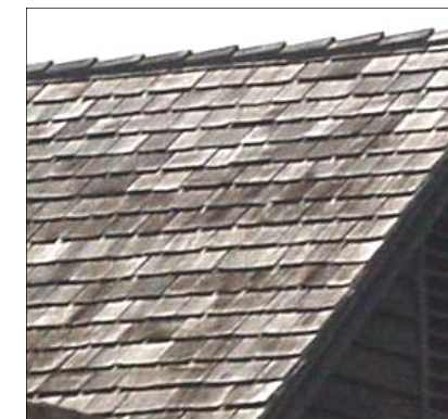
Shake or Shingle Roof
