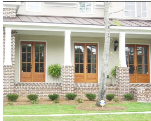
Square Tapered Columns on Brick Piers
