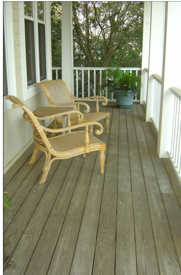
Treated Wood Floor (note: shallow porch)
