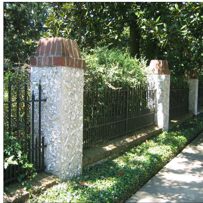
Wrought Iron Fence with Tabby Pillars
