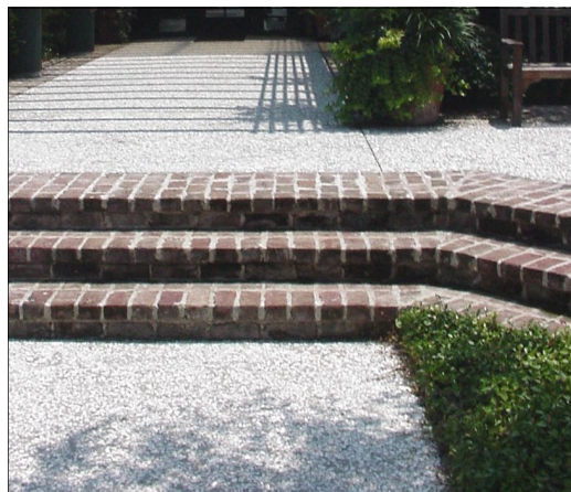
Aggregate Concrete w/ Brick Stairs
