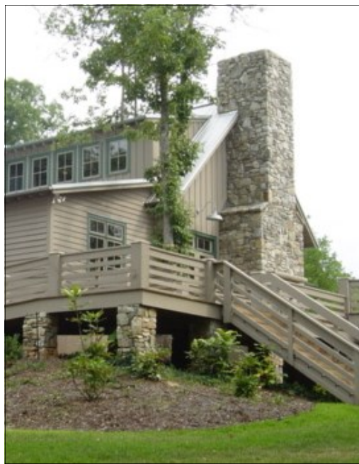
Stone Chimney and Foundation
