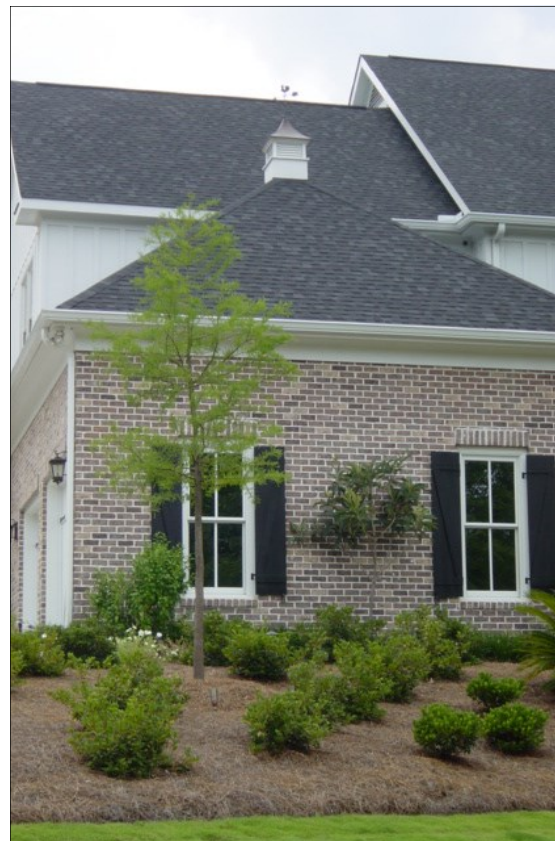
Brick with White Mortar
