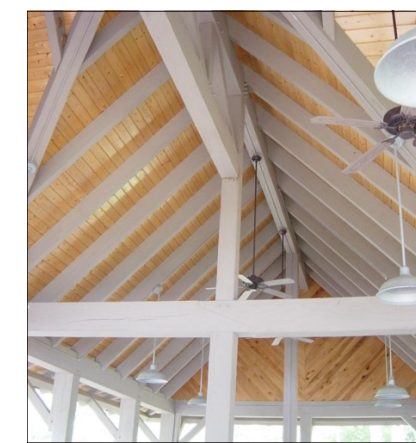
Exposed Roof Framing
