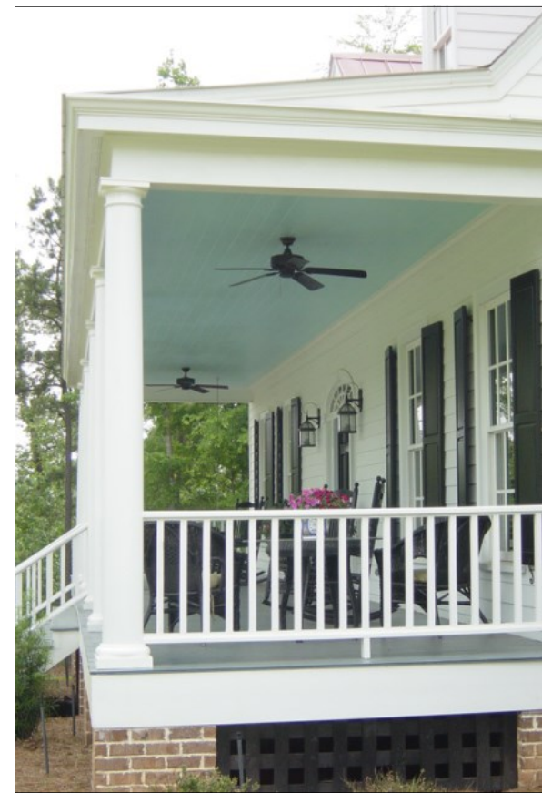
Painted Ceiling and Floor
