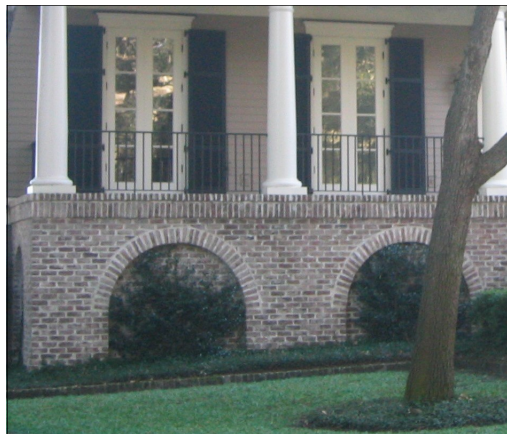
Brick Foundation with Arched Detail
