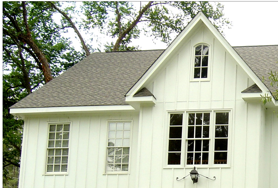
Board and Batten
