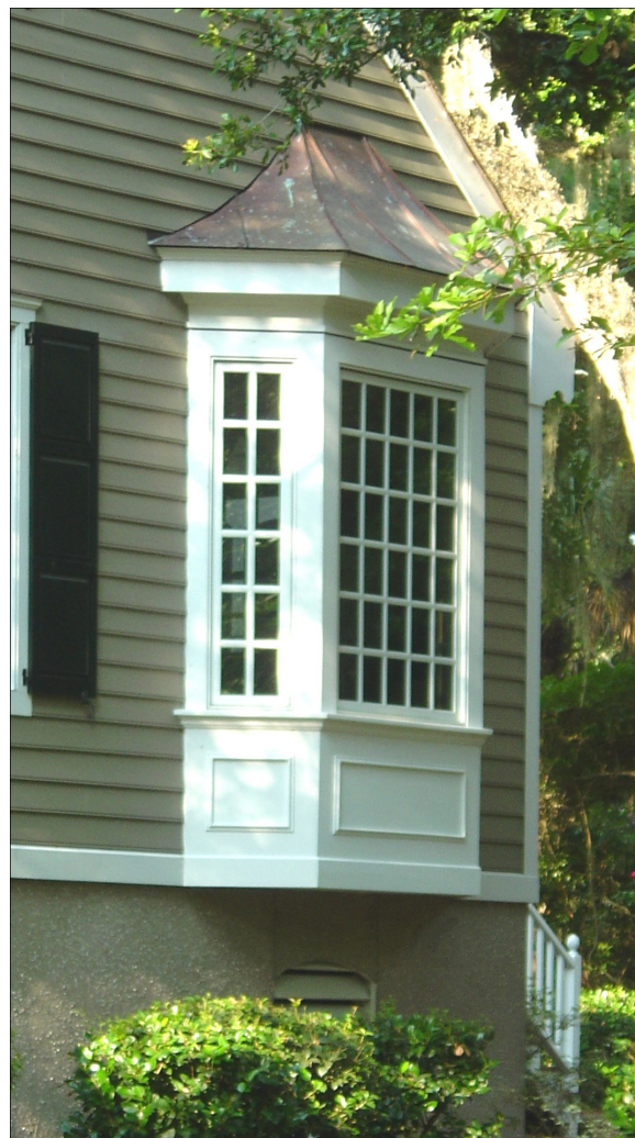
Bay Window with Copper Eave
