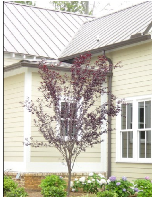
Hand-Crimped Standing Seam Roof
