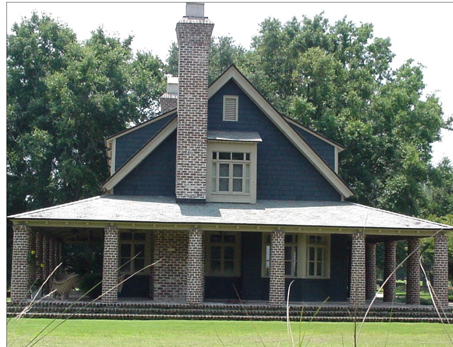
Brick Chimney and Foundation (Savannah grey brick with white mortar)
