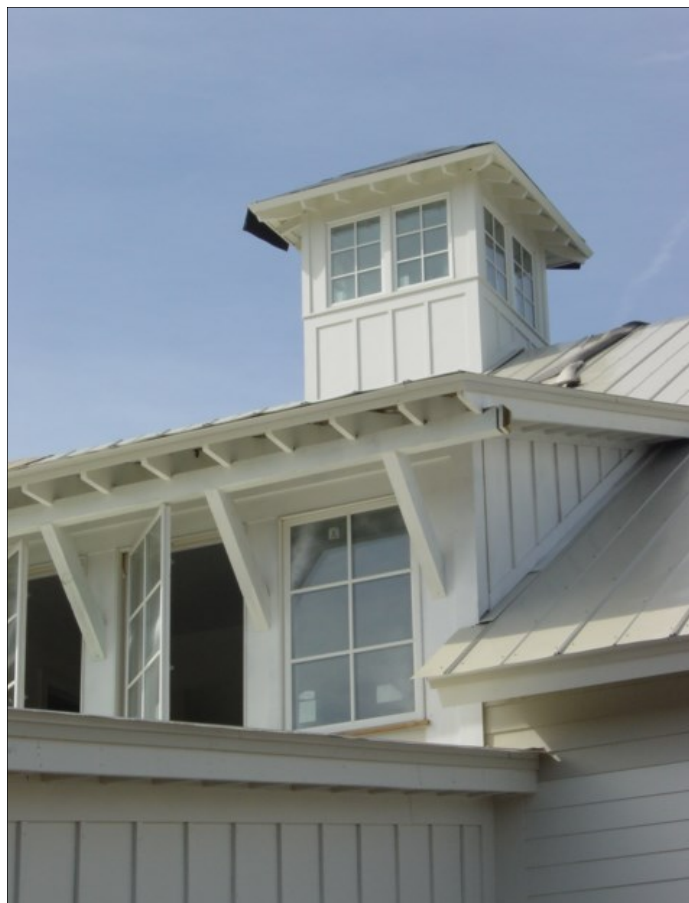
Exposed Rafter Tails with Bracketed Cornice
